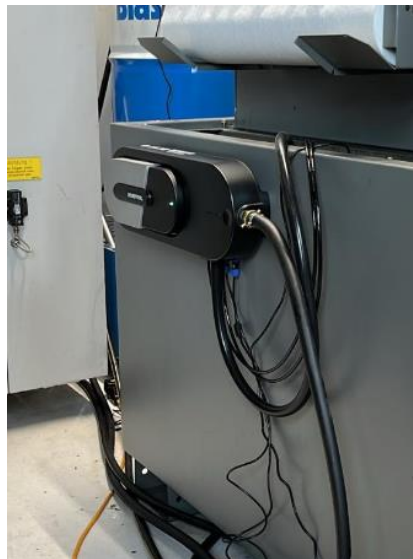
Horizontal on tank
